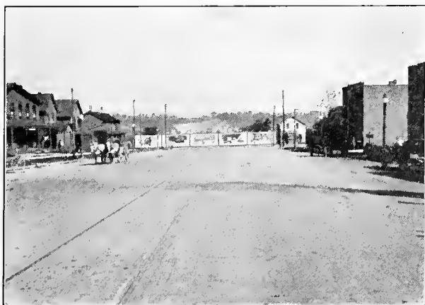
Present termination of Main Street, soon to be given a dignified and adequate outlet by the new Viaduct to North Hill
